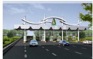
Highway Toll Station
